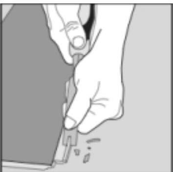
Fig 13. Horizontal installation (where angling is not possible). Cut off the locking element by using for example a chisel.
