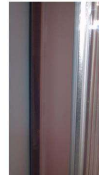
Step 3 – Remove protective film from the edge of the closure strip and apply ¾" x ¾" soft foam gasket material.
