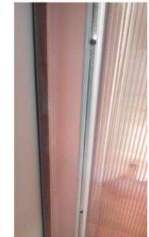
Step 7 – Install screws through the closure strip into the sheet metal strip. DO NOT SCREW INTO THE ALUMINUM. When you remove the closure strips the polyethylene double sided tape will peel off of the aluminum without leaving any residue.
