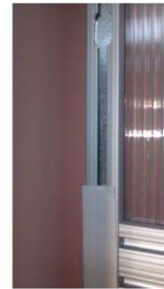
Step 2 – Apply double sided polyethylene tape to the face of the panel side rail. DO NOT USE FOAM TAPE.
