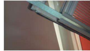
Step 1 – Insert ½" sheet metal backer strips into the panel's aluminum side as shown.
